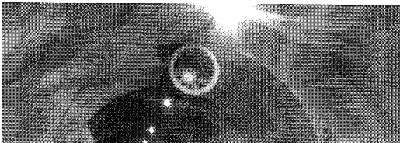
Sl.10 – Ventilator u tunelu
